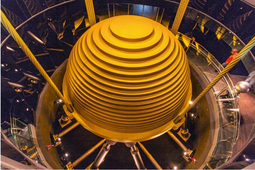
Fig. 18.12 TMD inside at Taipei 101
