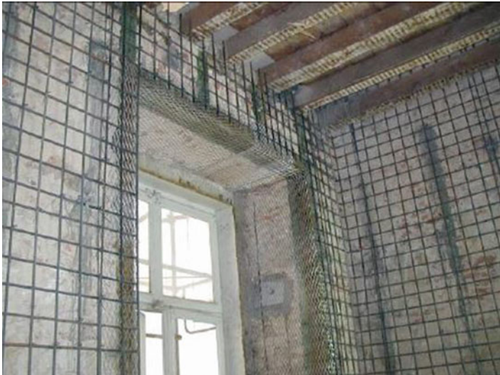
Fig. 20.72 Application of the welded grid from the inside
