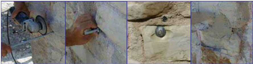
Fig. 20.63 Phases of laying the connectors
