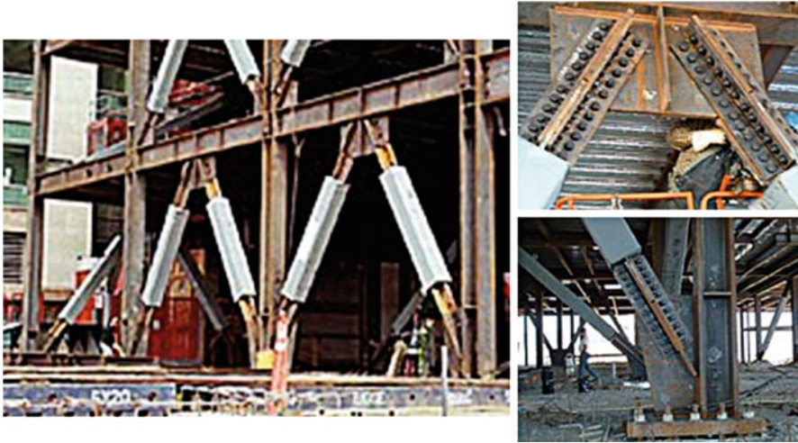
Fig. 17.15 Example of BRB dampers implementation
