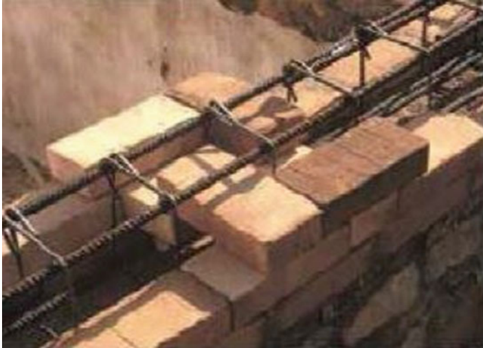
Fig. 20.55 Example of reinforced masonry top ring beam
