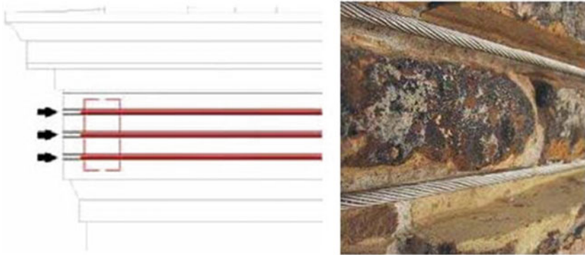
Fig. 20.53 Example of steel strand hoops
