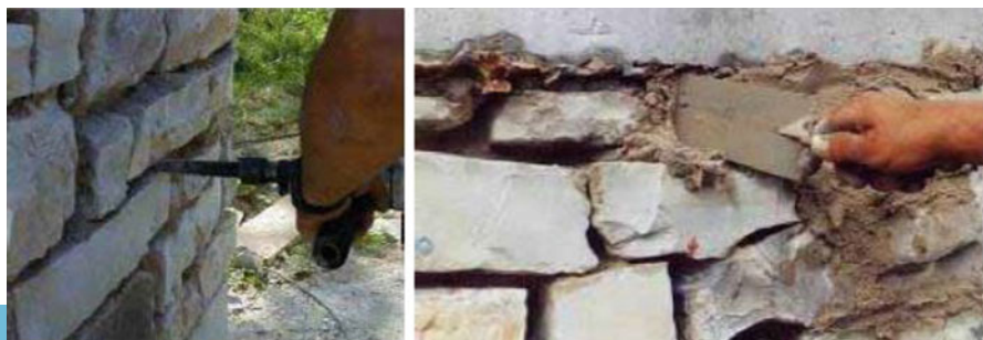
Fig. 20.70 Execution phases of the repointing intervention
