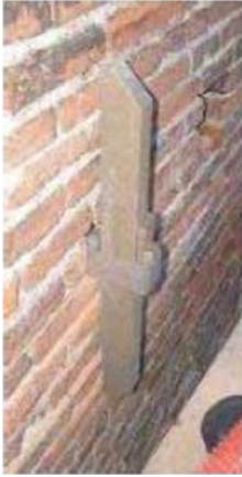
Fig. 20.49 Elements constituting a tie bar
