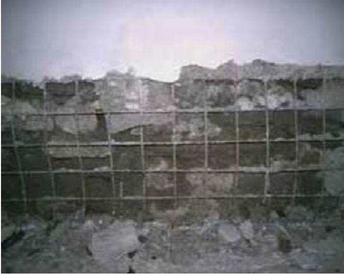
Fig. 20.73 Degradation of the reinforced plaster due to a lack of connection of the welded grid to the wall
