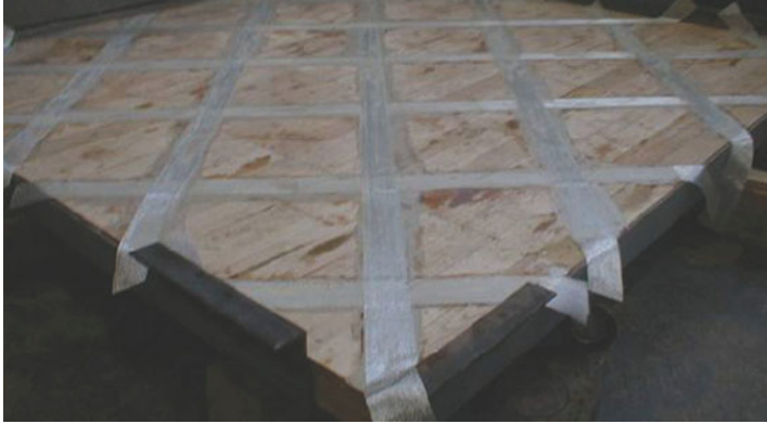
Fig. 20.60 Application of FRP stripes at the extrados
