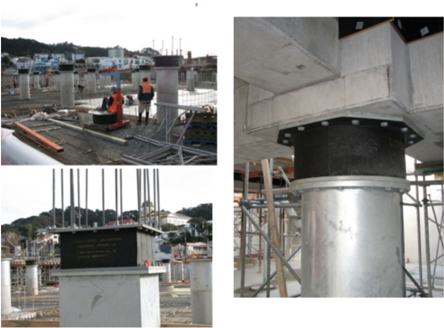
Fig. 19.26 Installation of isolator in Wellington Hospital (new building), New Zealand
