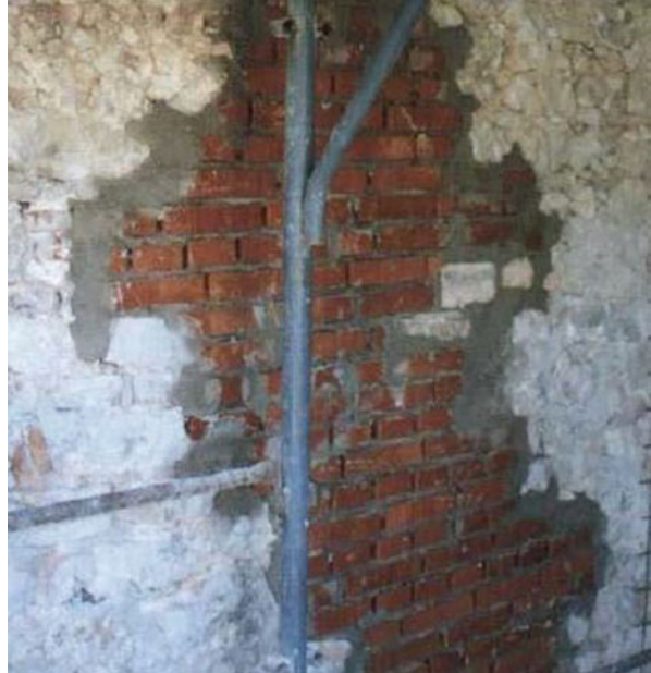
Fig. 20.62 Example of patching
